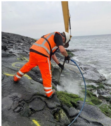
Figure 20. Pretreating the construction area by removing algae.
