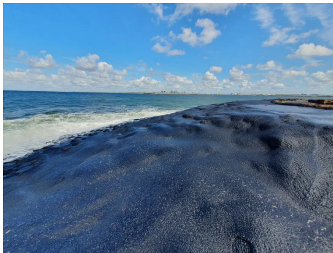
Figure 11. Photo of the repair in 2023 with the smooth asphalt top.
