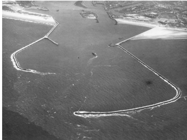
Figure 3. Photo of the breakwaters, on the right the longer southern breakwater, left, the northern breakwater.
