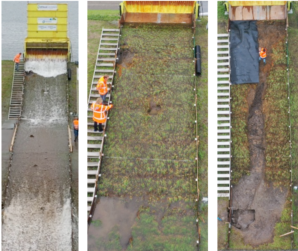
Figure 10. Instant development of initial damage half way the upper slope by one wave. The remains of the grass cover and clay sediment is visible on berm and down slope (left). Situation of failed grass cover (a hole in de middle of the test section with a depth of about 0.3 m) after 4 hours of 50 l/s per m with the sea/lake regime (middle). Failure of the geometrical transition (lower part of the picture) after the full test with the sea/lake regime and gully development in the boulder clay underlayer on the slope (right).
