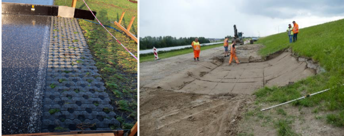
Figure 3. Concrete tiles with roughness in order to cancel the roughness effect at the location of the grass transition (left). Mixed-in-place solution at the geometrical transition (right).
