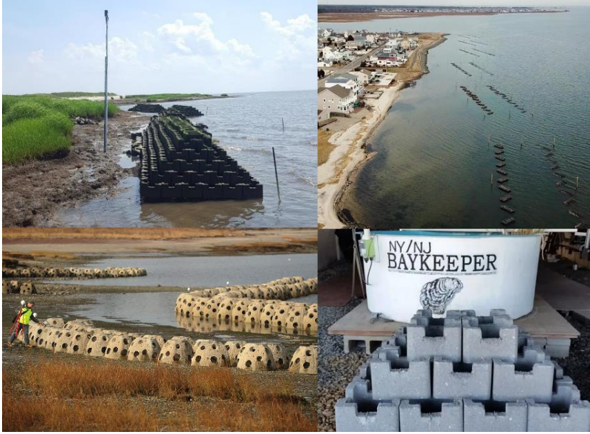
Figure 1. Images of the structures located all four sites, from the top left counterclockwise, Gandys Beach oyster castles, Forked River gabion baskets, Stratford Point reef balls, and Naval Weapon Station Earle oyster castles.
