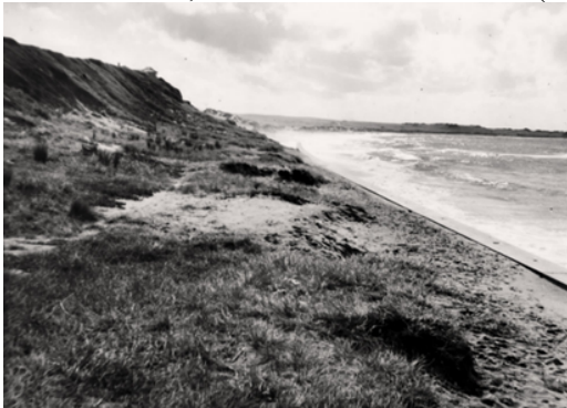
Figure 4. North Cronulla seawall in 1949
