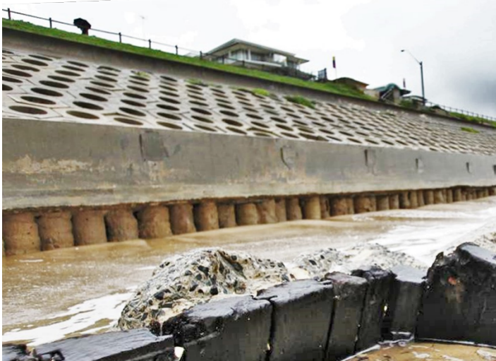
Figure 12. Contiguous pile wall after completion: note the pile gaps
