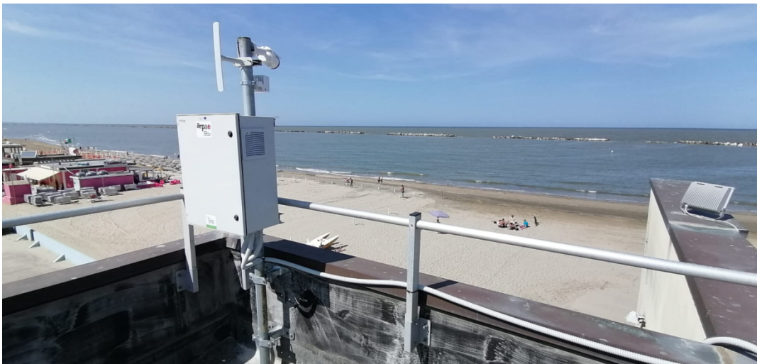
Figure 2. Webcam installed in Valverde (FC).
