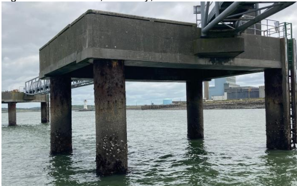
Figure 2 Mooring Dolphin, Shannon Estuary, Ireland
