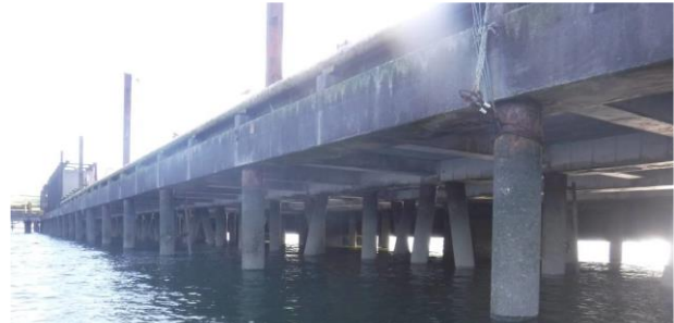
Figure 3 - RC Jetty on steel Piles, Cork Harbour, Ireland
