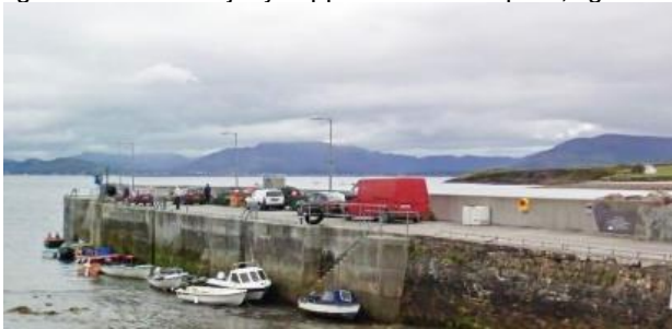
Figure 1 - RC Pier, Co Kerry, Ireland
