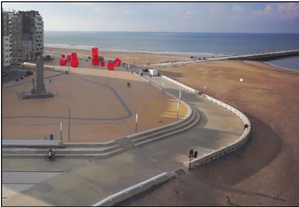
Figure 1 - sea dike with stilling wave basin at Ostend city
