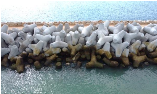
Figure 1 -Tetrapods in the Port of Molfetta (Italy). Source: Acquatecno Srl.
