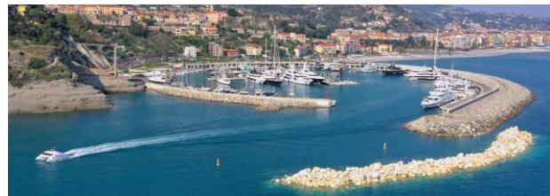
Figure 7 - Picture of the low-crested barrier realized to mitigate the wave agitation issue
