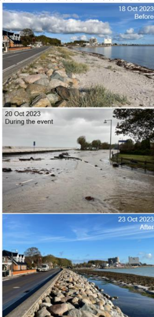
Figure 2: Pre- and post-storm conditions showing the impact along the nourished stretch of coast. Photo: Anna Adell and Klaus Roenholt.
