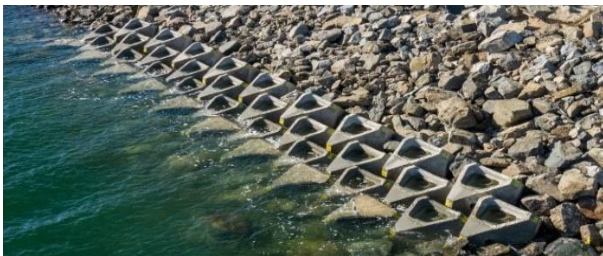
Figure 1. Coastallock armour units in the San Diego Port
