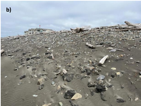
Figure 1 - Schematic profile of a dynamic cobble revetment showing how aeolian sediment transport might alter the roughness and porosity of the structure. b) Example of infilling after aeolian sediment transport on an engineered dynamic cobble revetment in Westport, Washington, USA (Photo: Hailey Bond).
