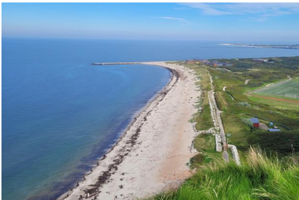
Figure 1 - Investigated northeastern dike section on the German island Helgoland (view looking east).
