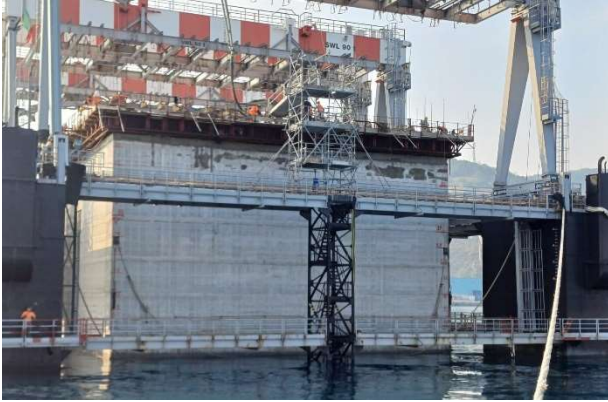
Figure 4 - Caissons construction on Company floating dock
