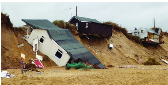
Figure 6 - Buildings collapsed after coastal erosion in Hemsby, UK in 2013 (Gray & Crofts (2022).
