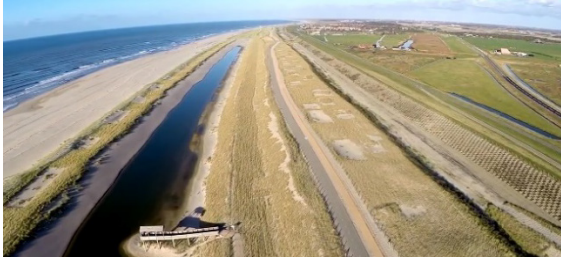
Figure 4 - Dunes created in front of the Hondsbossche sea dike (NL) to improve its safety level (HHNK, 2017)
