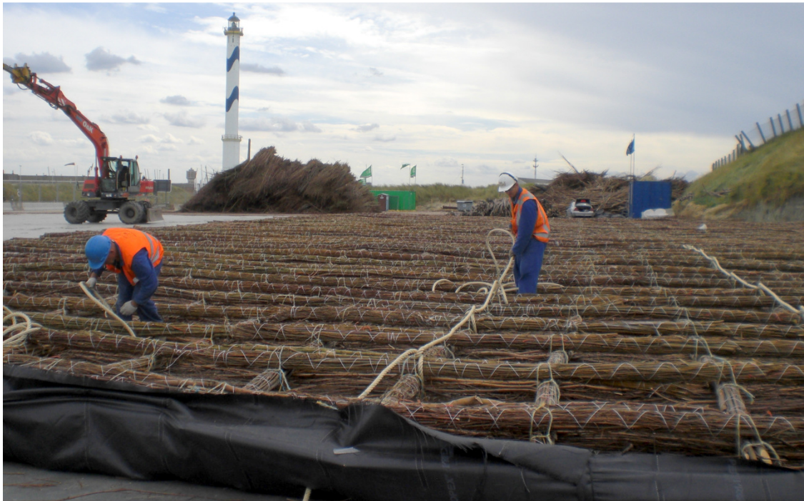
Figure 18. Willow mattress ready to be towed into the sea
