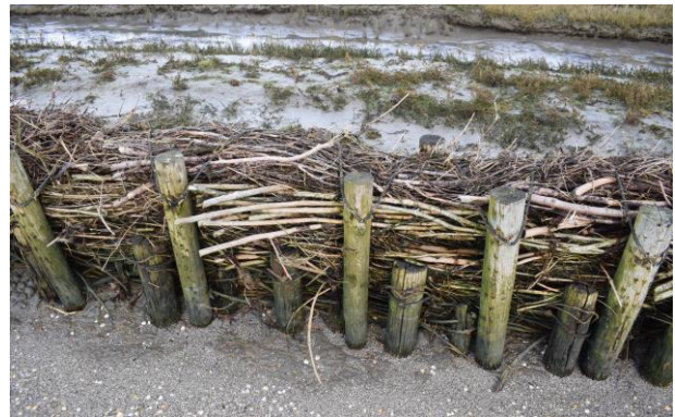
Figure 1: A brushwood groyne constructed within a salt marsh in Northern Germany
