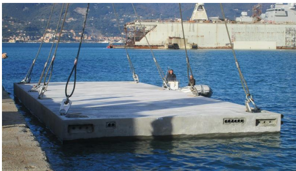
Figure 1. Example of a large floating breakwater unit installed at Port of La Spezia (photo courtesy of INGEMAR).
