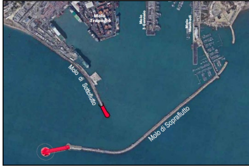
Figure 1 - The configuration of the Port of Salerno, red areas indicate the location of the works : the West breakwater was demolished for a length of about 100 m, while the East breakwater has been extended of about 180 m by adopting REWEC3 caissons
