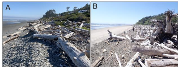
Figure 1 - Plat A: naturally occurring composite beach at Kalaloch, Washington with a cobble berm backing a sandy foreshore; Plat B: constructed dynamic revetment at North Cove, Washington.
