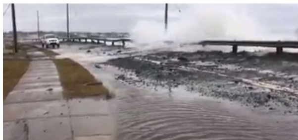
Figure 1 - Photo of site during storm event illustrating overtopping and flooding.
