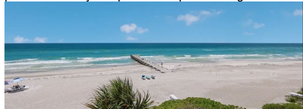
Figure 1. Longboat Key permeable adjustable groins a decade after initial construction, note the permeability of the structure allows for a subtle shoreline signature compared to traditional groins.
