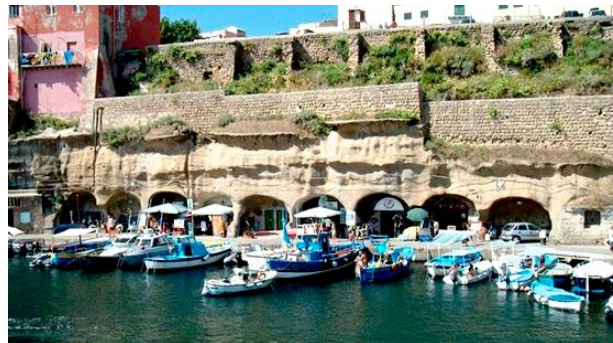
Figure 4 - Rock carved port storage caves
