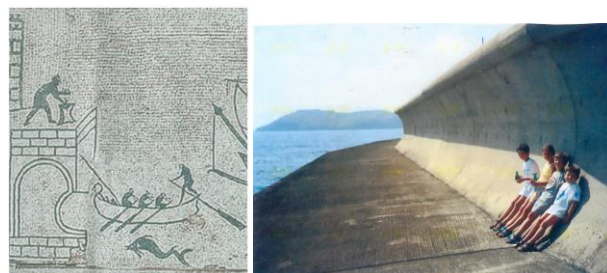
Figure 7 - Curved set-back wall in old mosaic and in the modern caisson breakwater under construction (1992).
