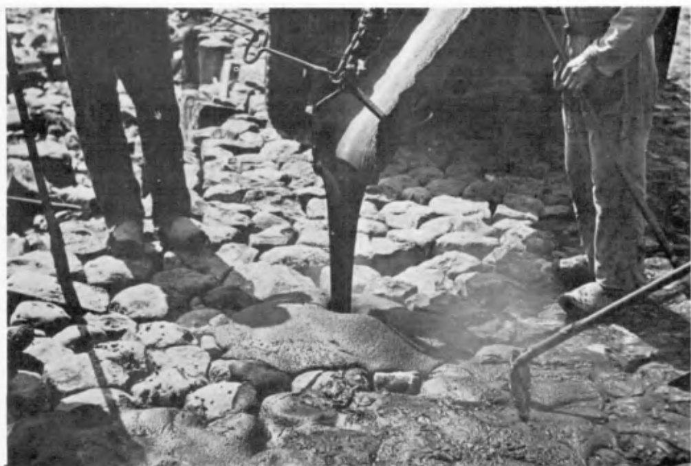
Photo 1. Asphalt grouting. (Copyright L. Spronk, Domburg, Holland)
