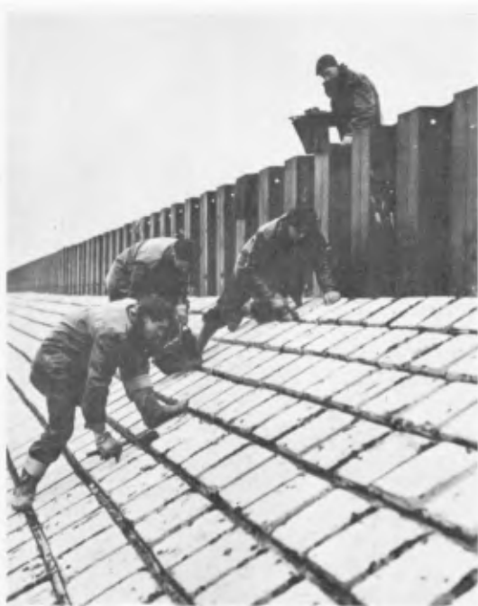
Photo 2. Asphalt jointing (Photo by courtesy of the Chief Engineer - Essex River Board).
