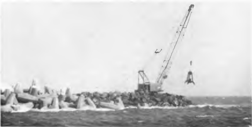
Fig. 6 Breakwater under construction
