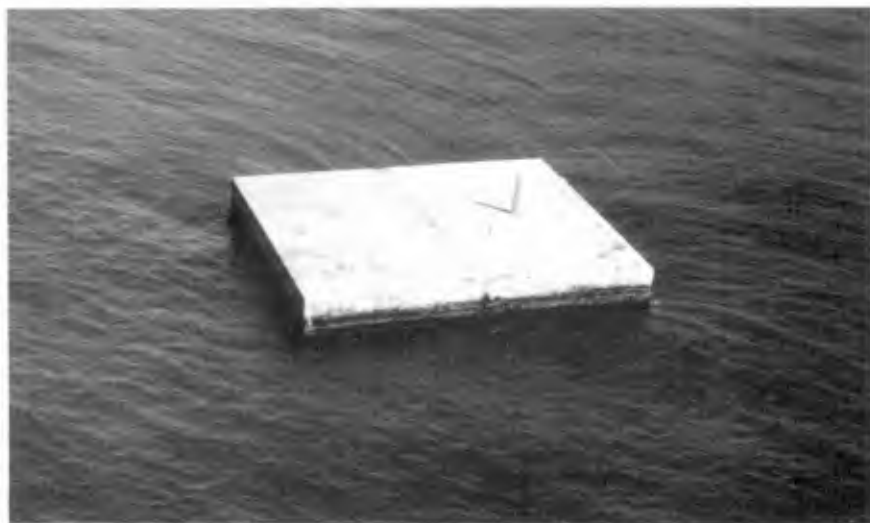
Fig. 10 Test breakwater at Tomakomai Port
