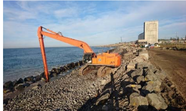
Figure 1: East London Foreshore Revetment during construction
