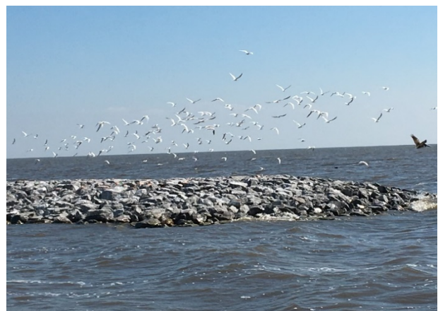
Figure 2 - Phase 1 Living Shoreline Breakwater
