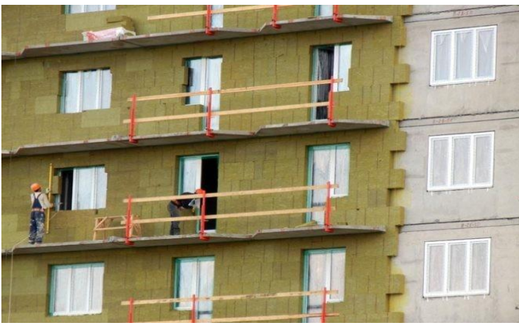
Picture 1. The process of using basalt fiber mats in buildings
