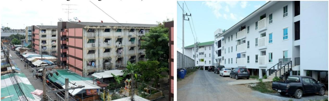
Figure 3. Public housing of National Housing Authority in Bangkok (left) and CODI Pathum Thani Model, relocated community in Pathum Thani, Thailand (right).
