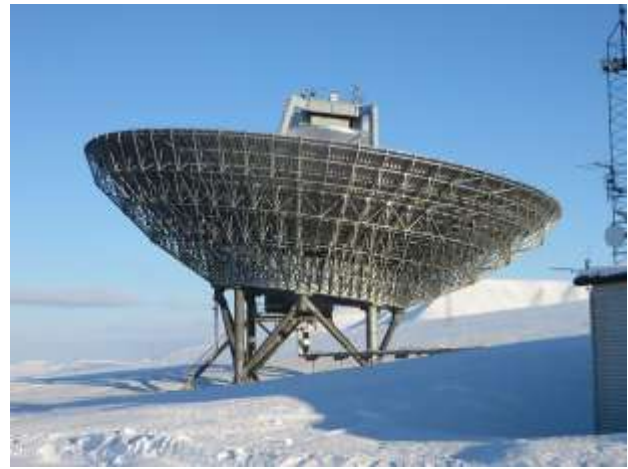
Figure 1. Fixed 42 m dish of the EISCAT Svalbard Radar. From EISCAT, 2015
