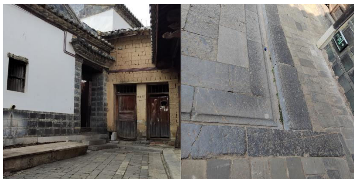
a. General first interior view
