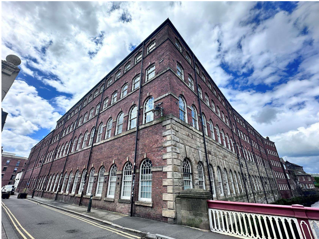
Figure 8. Cornish Place Works
