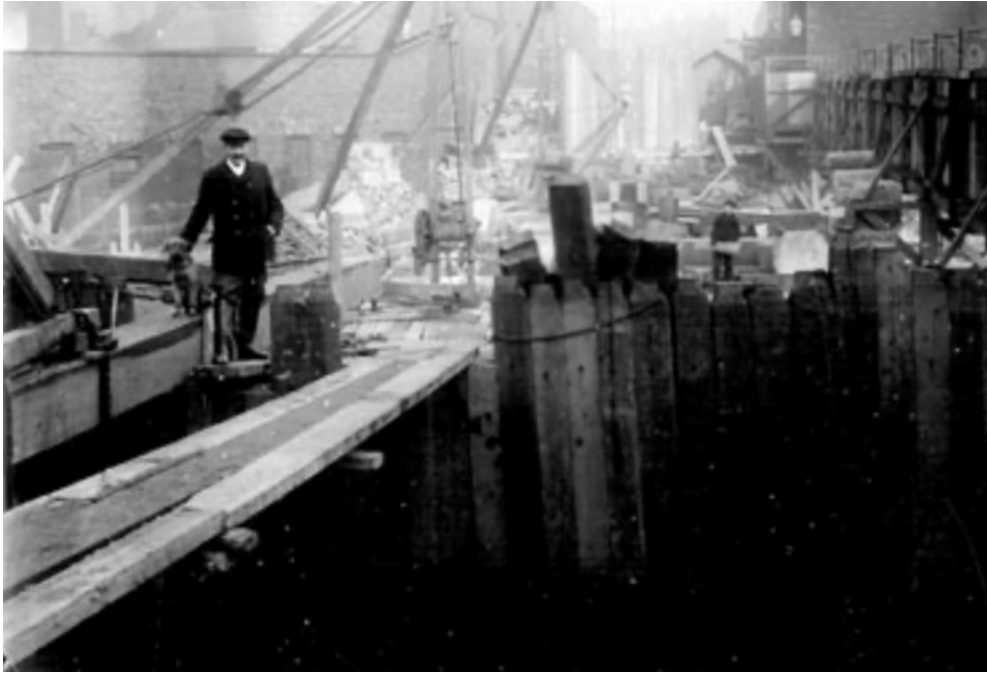
Figure 5. Re-building of Ball Street Bridge (Picture Sheffield, 1900-1919)
