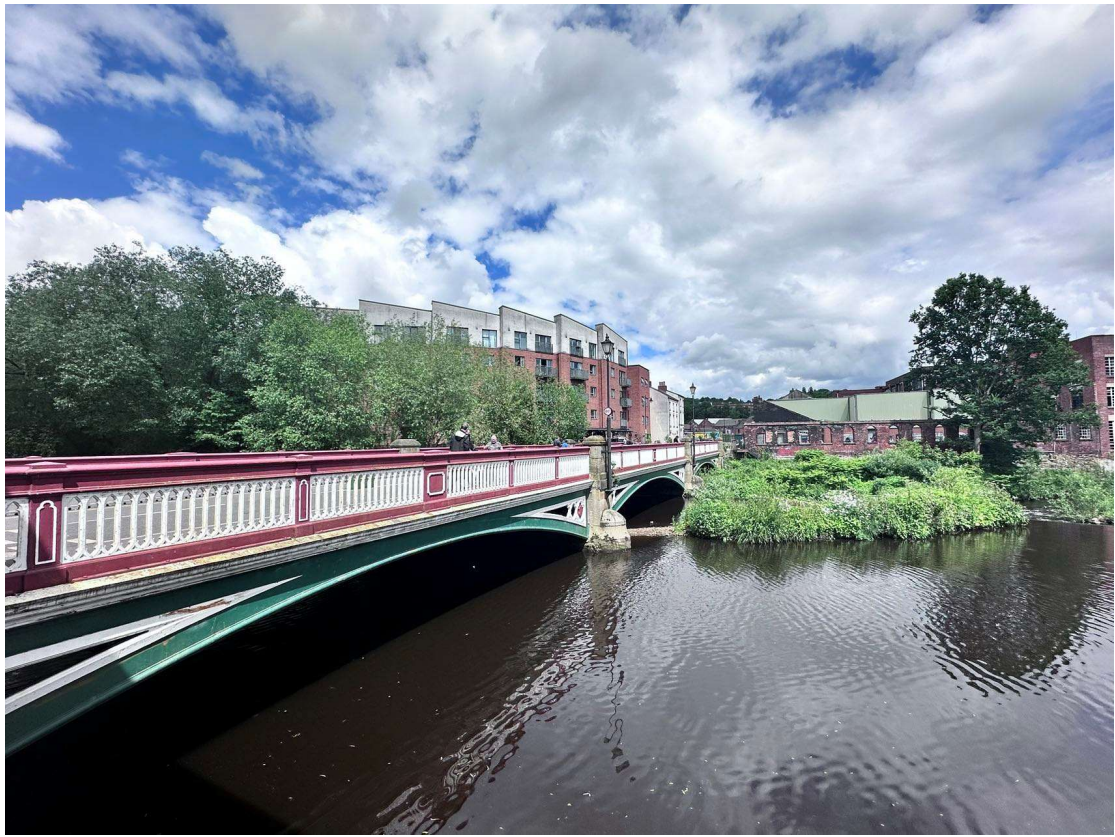
Figure 3. Ball Street Bridge
