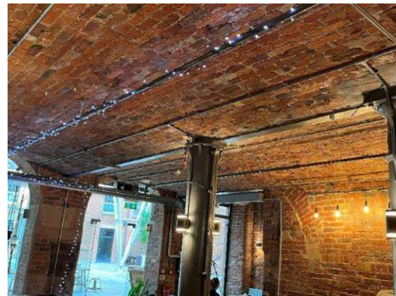
Figure 4. The Ceiling Structure of Royal Mill. Photo taken by author
