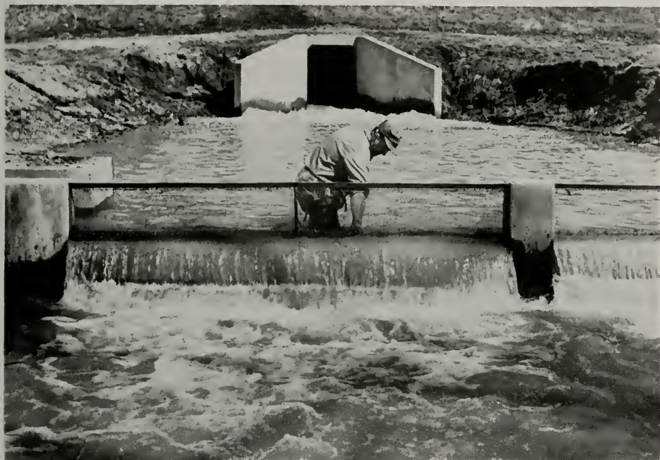
Fig. 9.—Improved type of fish screen used in draining censuses. A permanent screen was built below the outlet of Ridge Lake in 1948. It consisted of a wide concrete base, wing walls, and a center post double slotted to hold removable screen frames and planks. Planks placed below the screen frames created a head of water in the basin between the outlet and the screen and reduced the water pressure on the screen if the latter became partially clogged with debris. Screen frames could be raised for cleaning.
