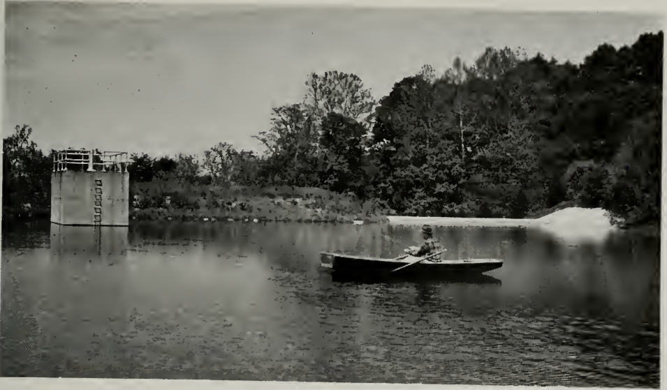
Fig. 2.—The dam, tower spillway (left), and surface spillway (right) as seen from the surface of Ridge Lake.
