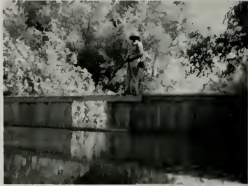
Fig. 33. —Small dam constructed at outlet of lake. The lake shown here is fed by springs; closing of the gate in the hunting season will flood the area.
