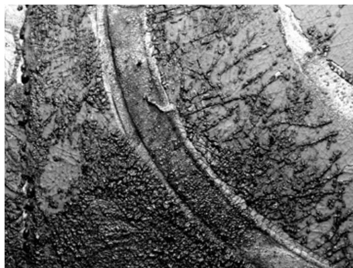
Figure 5: Restoration damage due to misuse of grease (Moritzburg gilt leather, detail of tapestry in the Kurfürstenzimmer II)
