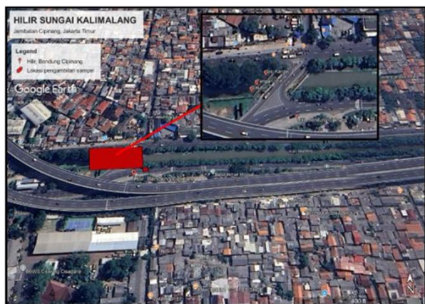
Figure 4 Jembatan Cipinang (Google Earth, 2025)
