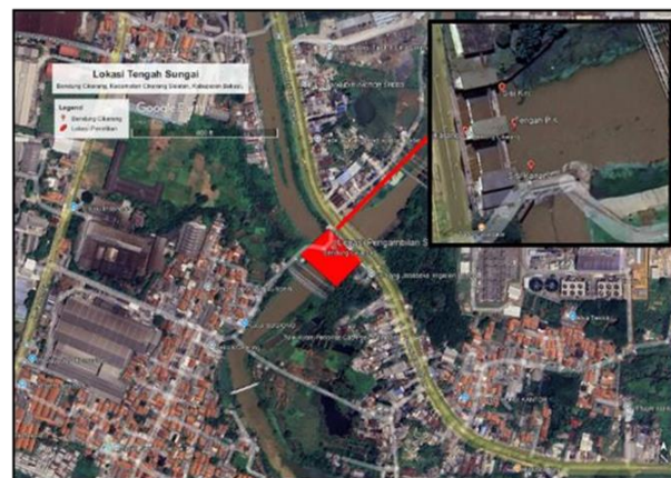
Figure 3 Cikarang Dam (Google Earth, 2025)
