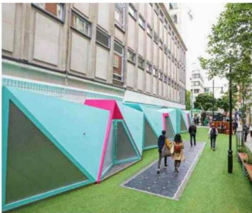
Figure 4: Bird street after renovation [8]
