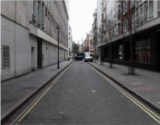
Figure 3: Bird street before renovation [8]
