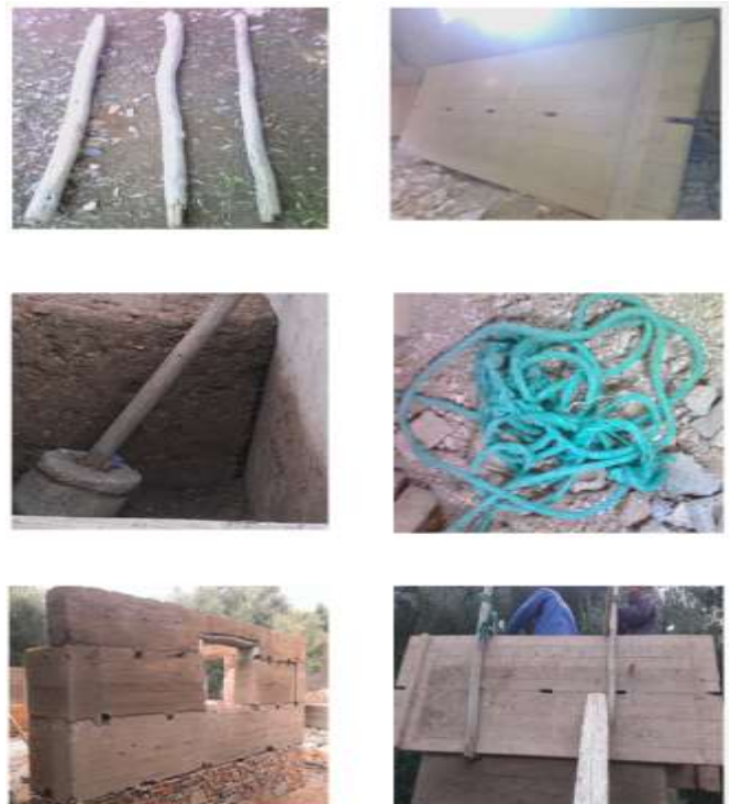
Figure 2: Traditional materials for rammed earth construction, Tiznit, Morocco
