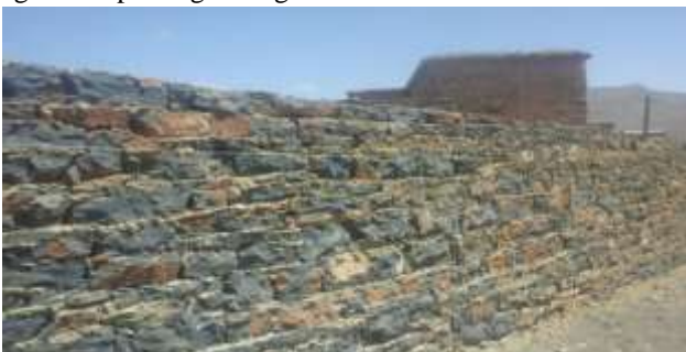
Figure 7: Traditional stone masonry, Morocco
