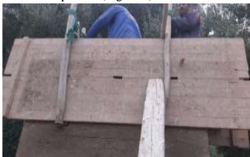
Figure 4: filling the mould of rammed earth, Tiznit Morocco
