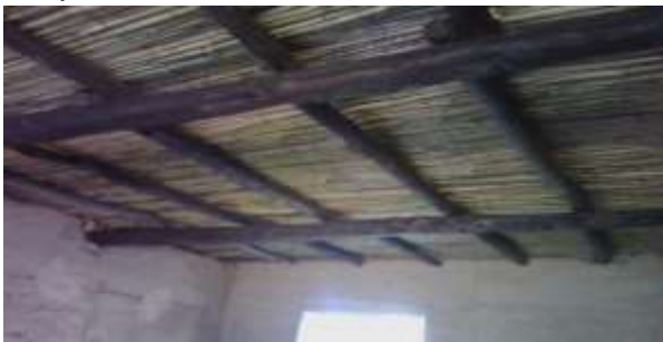
Figure13: Traditional wooden floor Tiznit, Morocco
