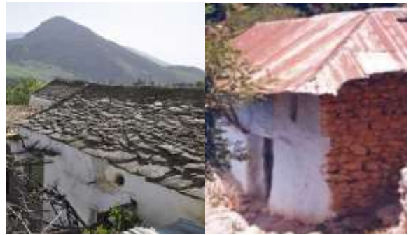
Figure 14: Roofing system based on earth, stone and wood (Mountainous area Morocco) [54].
