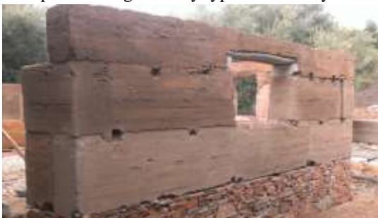
Figure 1: Raw earth wall, Tiznit Morocco
