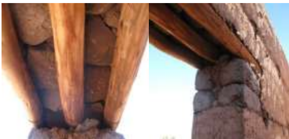
Figure12: Traditional wooden lintel, Tiznit, Morocco
