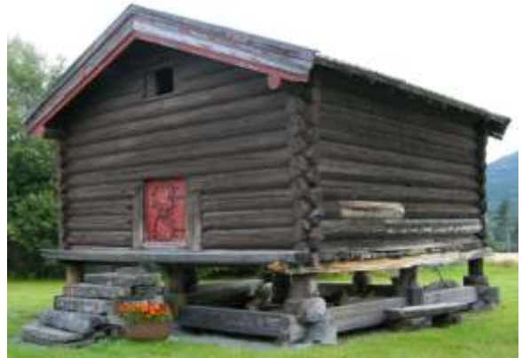
Figure 9: Stacked log loft (1193), Rilag, NORWAY [49]
