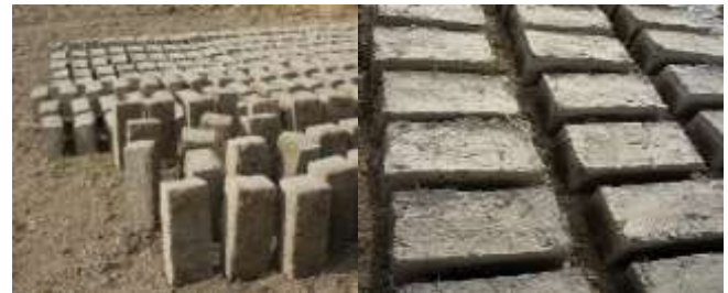
Figure 5: Adobe manufactured by traditional methods, Morocco
