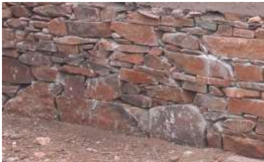
Figure 3: Stone base under the raw earth, Tiznit Morocco
