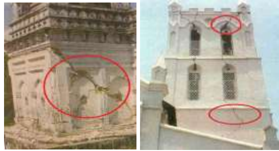
Fig. 2. Diagonal Cracking
