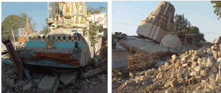
Fig. 1. Collapse of Structures
