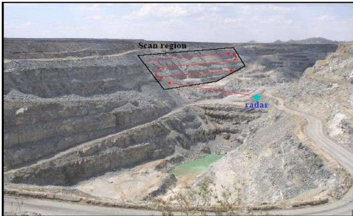
Figure 9 Radar-Based Monitoring of Slope Stability in Open-Pit Mines
