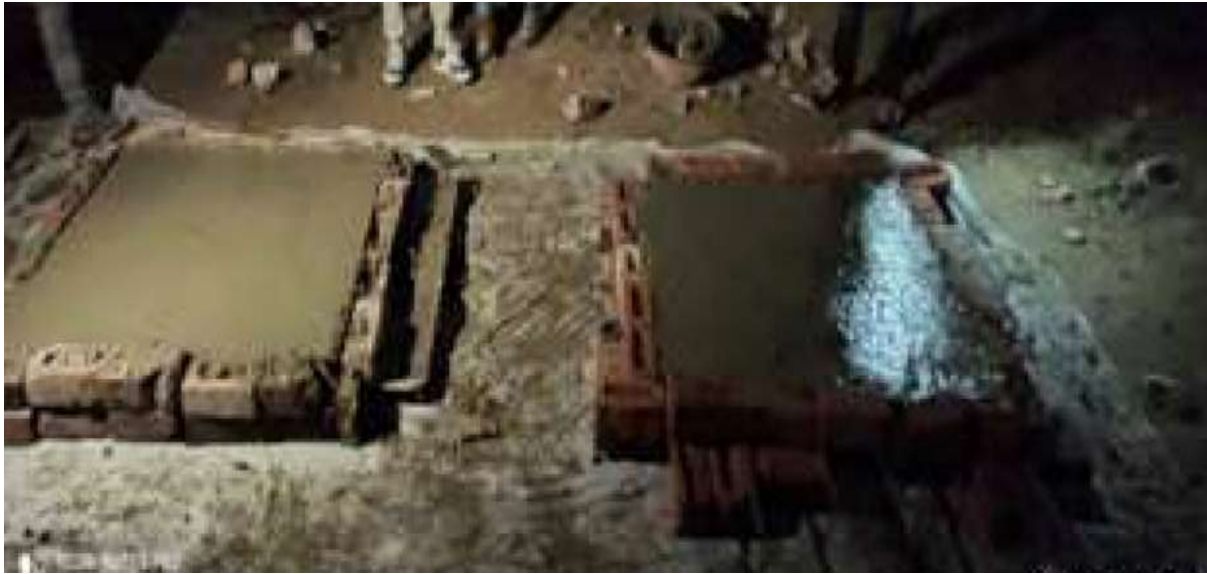
Figure: 1, Casting of slab Specimens
