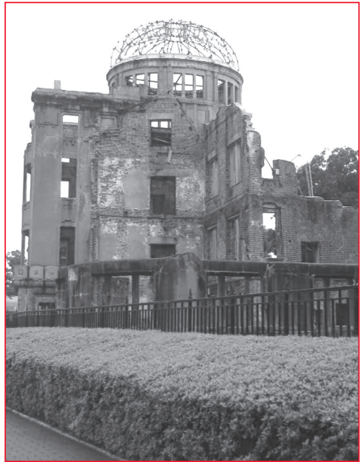
Figure 12– The “A-bomb building” as it appeared in July of 2019. Many Japanese would like to have this relic torn down since it is structurally dangerous and, understandably, is an unpleasant reminder of an event that they would rather forget. Photo by author.
