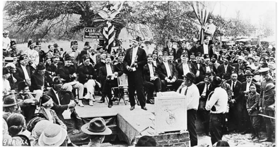
Figure 3. Laying of the cornerstone for the Shreveport Hospital
