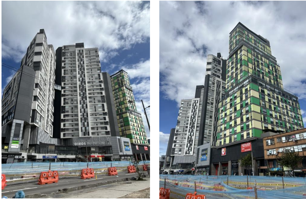
Figure 6. New developments on Caracas Avenue in front of the future elevated infrastructure of the First Line of the Metro Project of Bogota. Sources: Fieldwork visits in 2024
