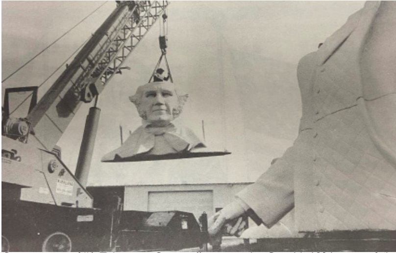
Construction of “A Tribute to Courage,” seen in the Oct. 16, 1994, issue of the Huntsville Item , retrieved from the SHSU Archives
