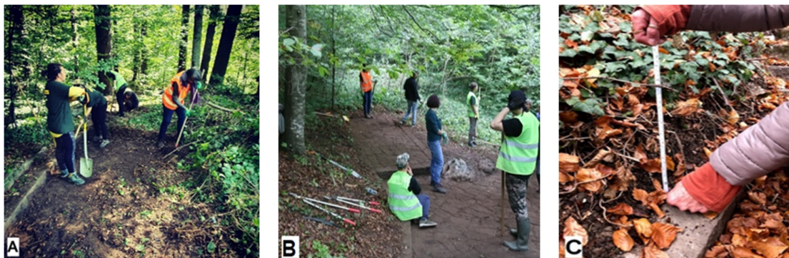
Figure 5. The new layer of soil (formed in decades of poorly maintenance) covering an alley (A) vegetation removal; (B) alley clean up; (C) layer of 25 cm, visible near the cleaned alley
