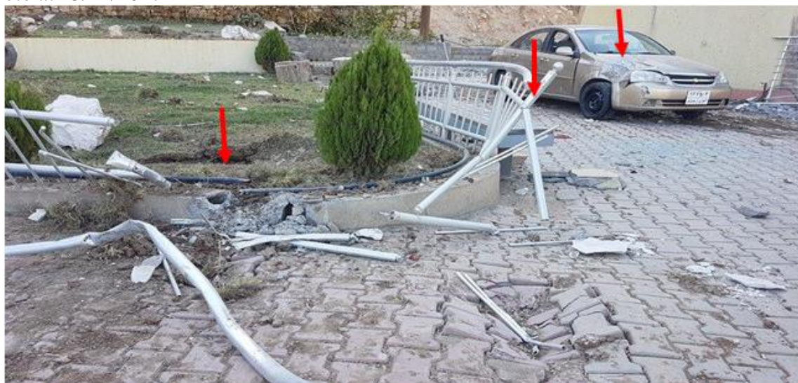
Figure 5. Fall down rocks in Zmnako mountain and demolition parks and breaking cars
