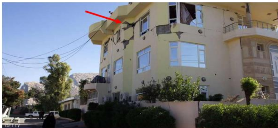
Figure 2. The folded and destroyed building faces by the earthquake
