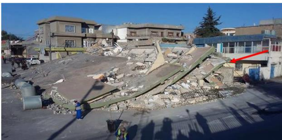
Figure 1. Collapse buildings by an earthquake in Darbandikhan town
