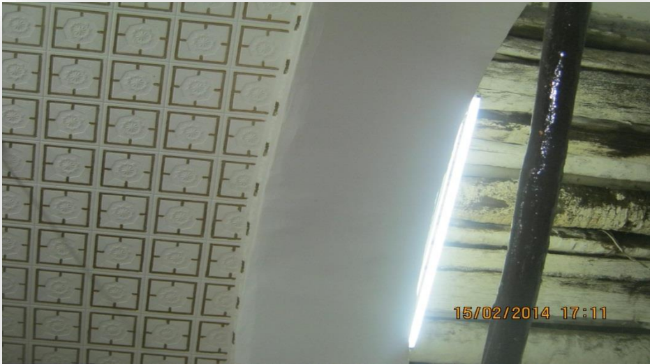
Photo 03 :Restoration with ciment and ceramic mosaics.The work of the researcher.
