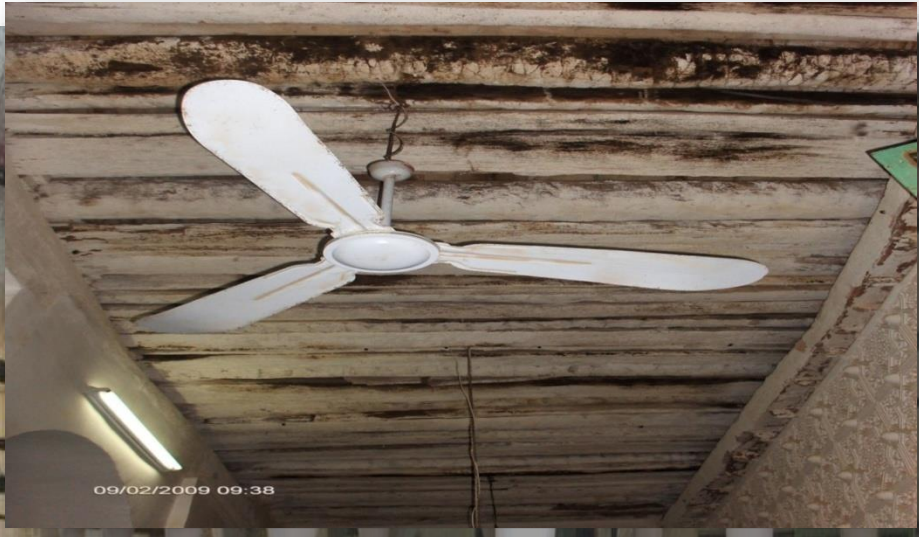
Photo01: the original roofing method.the work of the researche
