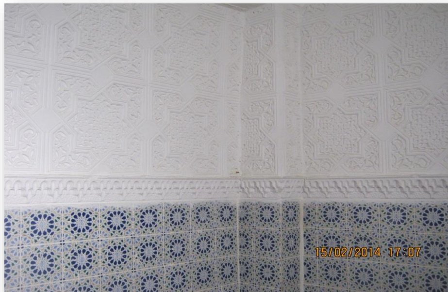
Photo 05 : Decorating with plaster on the walls.The work of the researcher.
